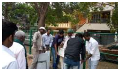
CONSTRUCTION OF WALKWAY 09-02-201
